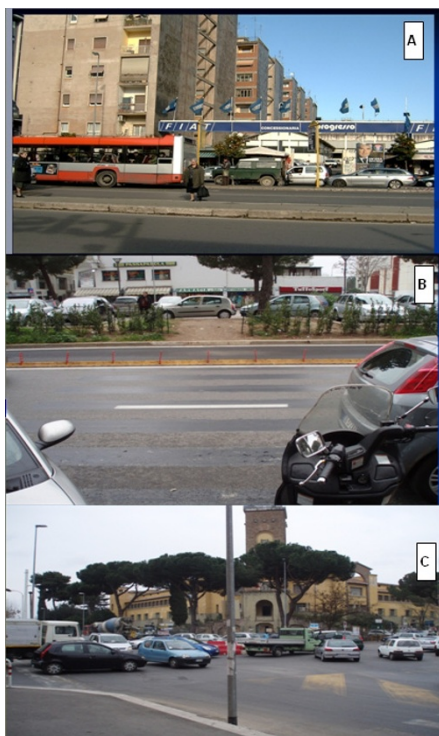
Figure 8 RTIs involving pedestrians – high risk roads. LHU Rome B year 2003. The picture shows a bus stop without any zebra crossing connecting the platforms and that the zebra crossing was removed, but the signs on the road pavement are still evident. The last picture (C) shows crowded crossing with poor traffic signs for both vehicles and pedestrians.
