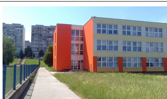
Figure 2 A typical elementary school within the typical neighborhood of housing estates. Note: The picture depicts a typical elementary school wedged into the fabric of a housing estate from the 1980s. Although the school building has been renovated, it still does not represent a truly inspiring environment for learning and play. Source: authors.
